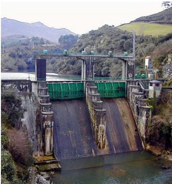
Fig. 9 The Palombera dam (23 m) has been blocking the passage of migratory fish in the River Nansa since 1949 (García de Leaniz et al., 1987; Serdio et al., 2001b). As its concession will soon come to an end, conservationists, scientists and anglers alike are campaigning for its decommissioning
